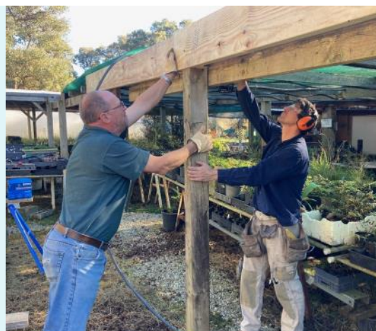
Kelvin and Jason fixing the beams.
